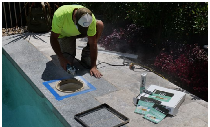
This retrofit took about 90 minutes. It all depends on the material to cut out and skill of the operator.
